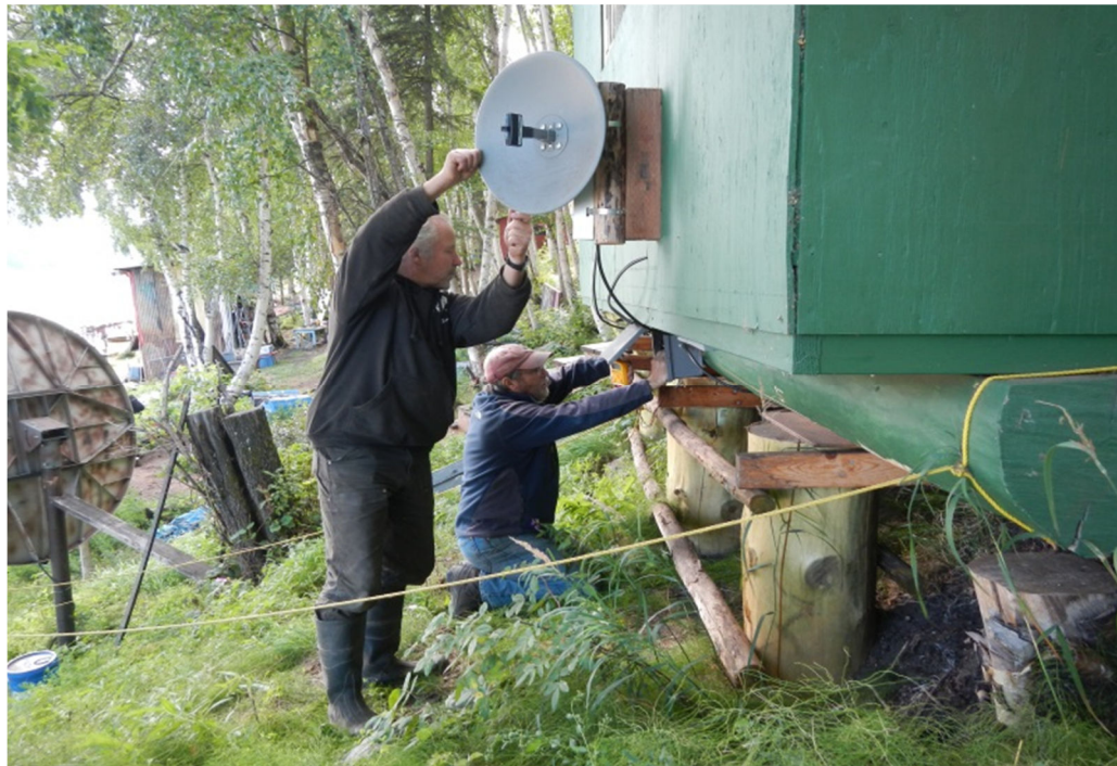
Stan Z. and Dave Daum (project partner) make fine tuning adjustments to fishwheel microwave receiver .
