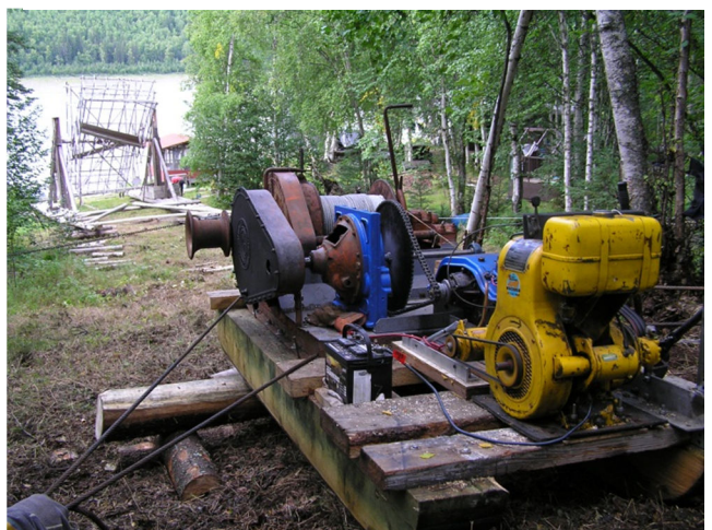
Winch used by project to move wheel in and out of water at Rapids
