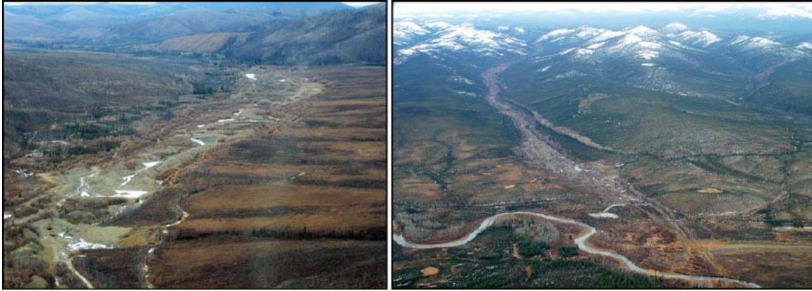
Figure 41. Heavily mined streambeds in Colorado (left image) and Ophir (right image) Creek valleys in the upper Innoko River drainage. Photos by R.J. Brown, USFWS.
