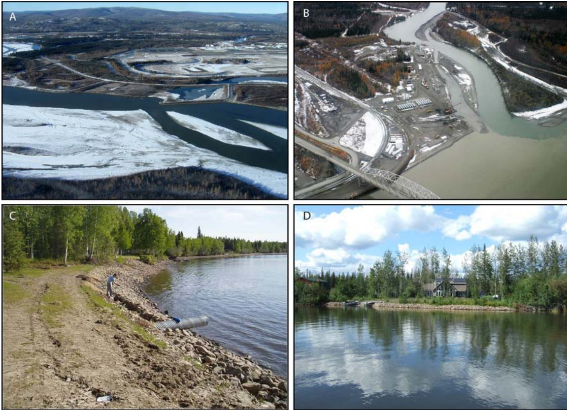
Figure 58. Four examples of large to small scale bank alterations that are common within the Tanana River drainage. A dike with J-shaped groins has been constructed between the Fairbanks International Airport and the Tanana River to slow erosion in that direction (A). It was recently discovered that this region of the river is a major spawning area for several whitefish species. The mouth of the Nenana River (B) is the upstream terminus of the freight hauling barges in the Yukon River system. As such, it is an industrial site with extensive bank stabilization in the docking area along the Tanana River frontage (the downstream edge of which is seen under the bridge in the lower left), and annual dredging of the Nenana River mouth for fill material and to support other barge activities in the area. Vegetation has been cut and boulders have been dumped along the banks of the lower Chena River to channelize the river course through the community of Fairbanks (C). Riverfronts have been cleared and banks have been stabilized with rocks in front of many riverfront houses in the Tanana River drainage (D). Photos by USFWS staff.
