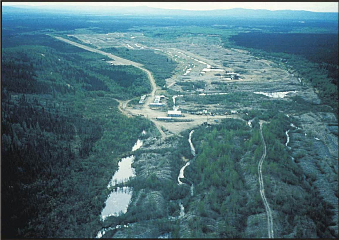
Figure 14. An aerial image of the Bear Creek mine in the Hogatza River drainage, Yukon River basin. The streambed was mined with a large floating dredge, rerouting the stream course as necessary. Photo by USFWS staff.
