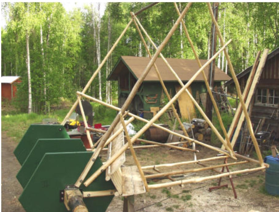
The baskets were built on the plates one at a time and then removed for transportation to the riverbank.
